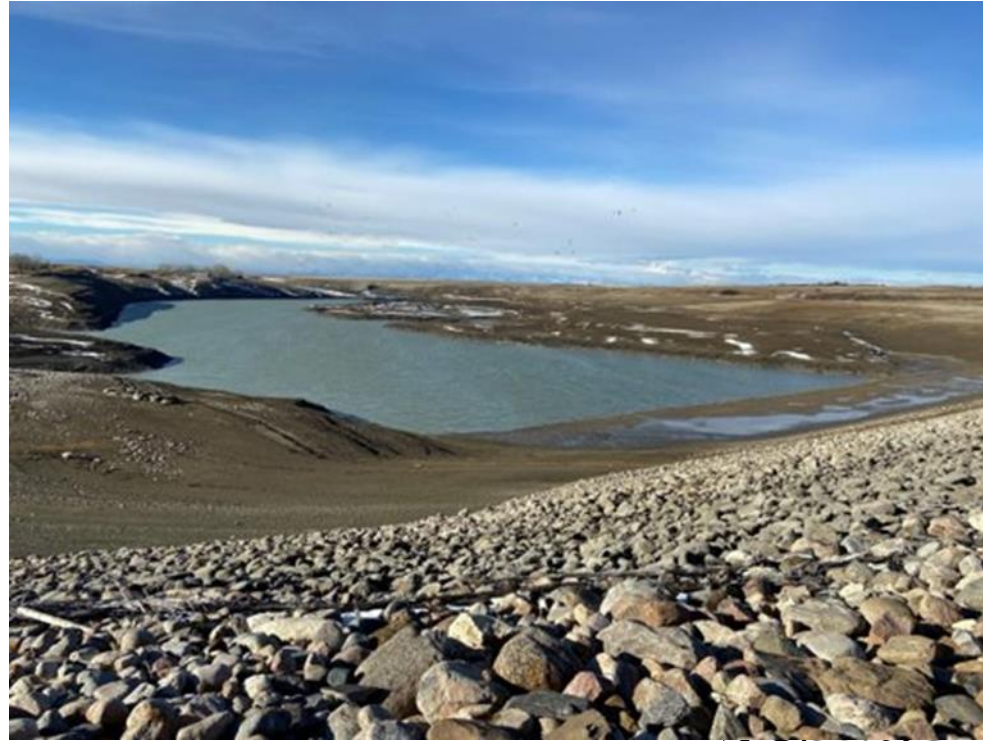
View from the top of the dam
