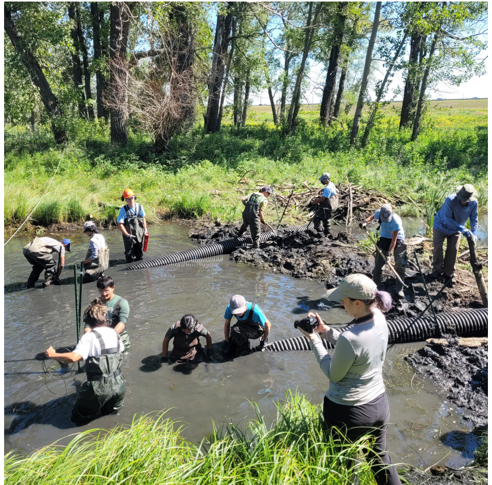
Pond leveler installation. Photo: The Friends of Fish Creek.
