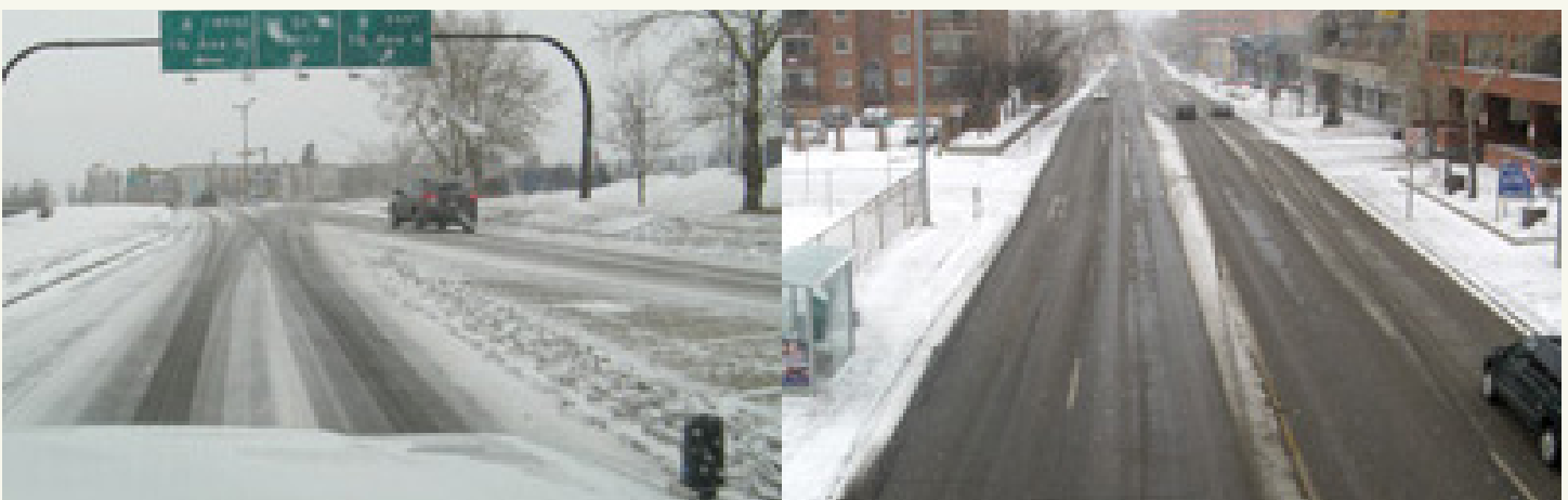
Before and after photo of de-iced roadways. The City of Calgary only uses sodium chloride and calcium chloride. Road salts used for snow and ice control may be solid or liquid brines. Photo: The City of Calgary.
