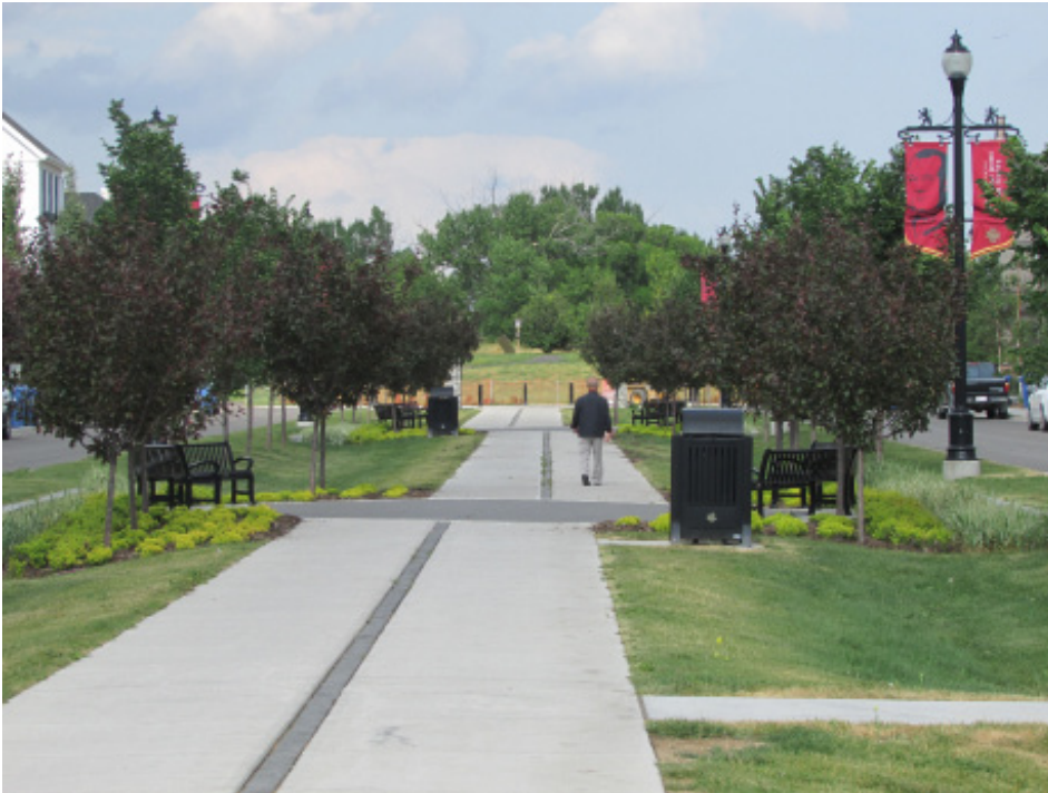
Infiltration trench and swale, Canada Lands Company's Currie Barracks redevelopment in Calgary. A gravel chamber overlain by a thin layer of absorptive soil and conventional sod replaces the storm sewer. Photo: Alberta Low Impact Development Partnership
