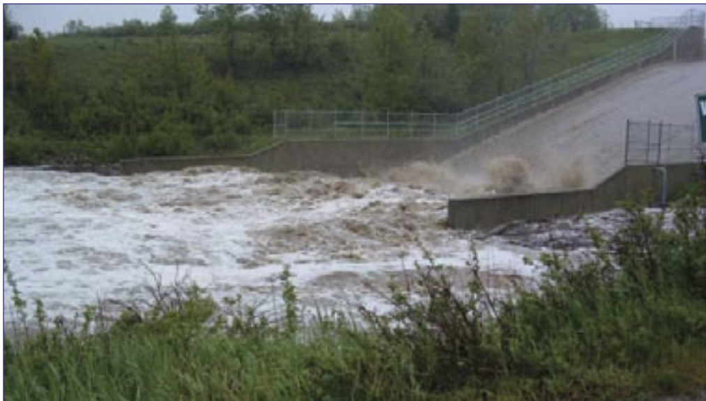
Chain Lakes spillway in flood. BRBC file photo
